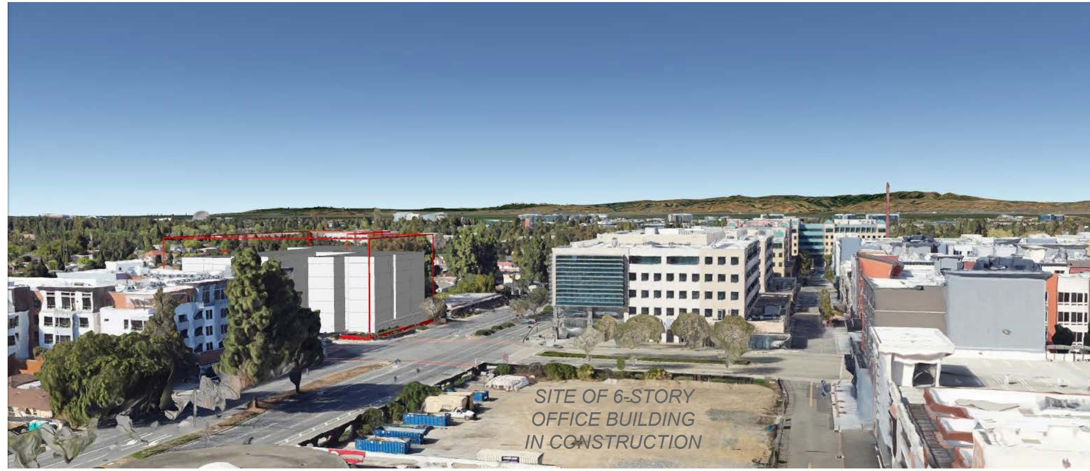
1a VIEW TOWARD NORTH FROM SOUTH MATHILDA AVENUE
