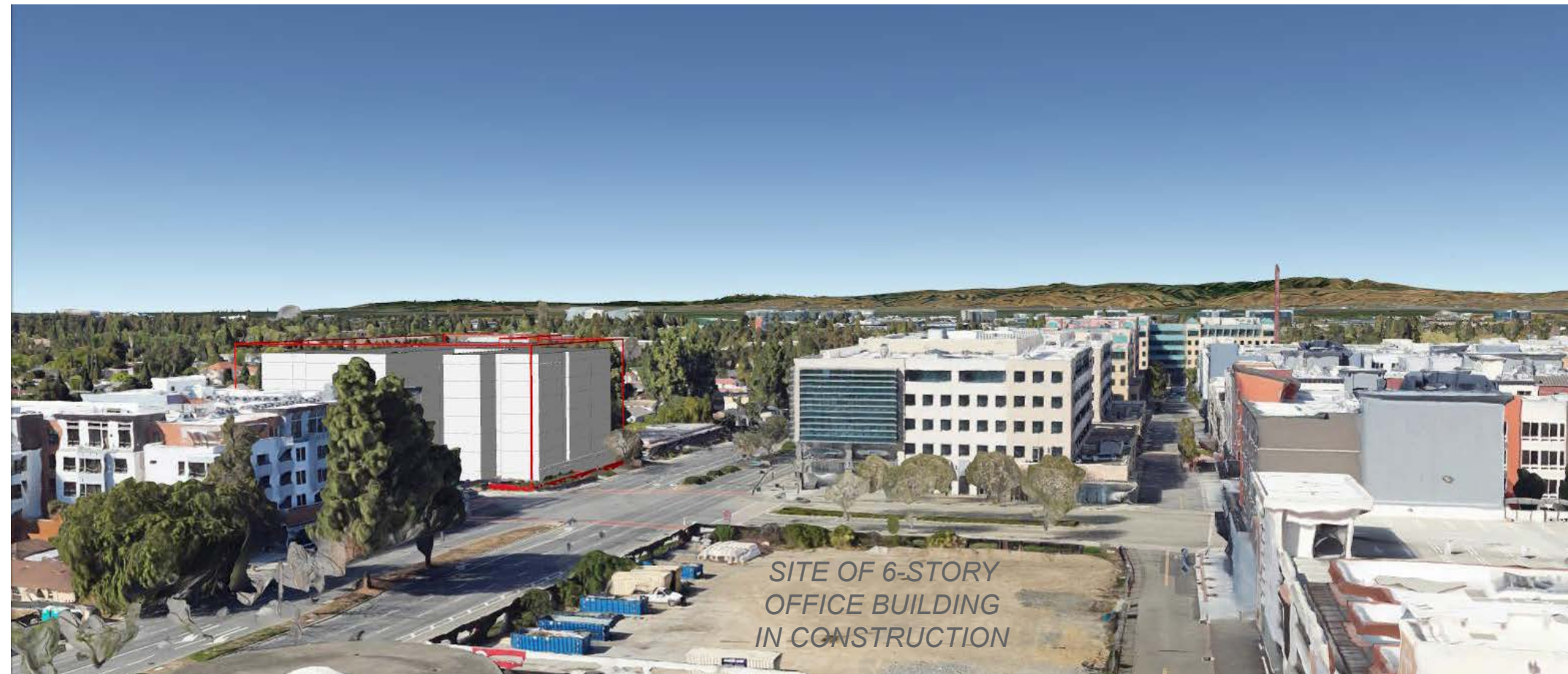
2a VIEW TOWARD NORTH FROM SOUTH MATHILDA AVENUE
